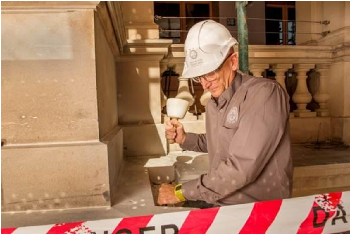
Pictured: Vince MacKenzie-Ross, Queensland Heritage Masonry. Image by Jeff Camden.
